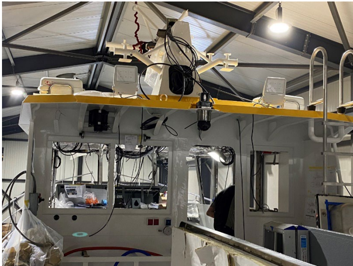
Superstructure view from the working deck, with the mast, deck lighting, life rafts, navigation lights and ladderway visible.
