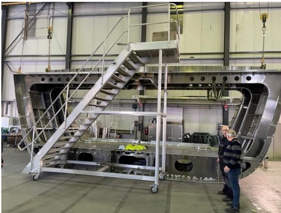
• Ring section 5, consisting of sections 350 and 450 is beginning to take shape.
