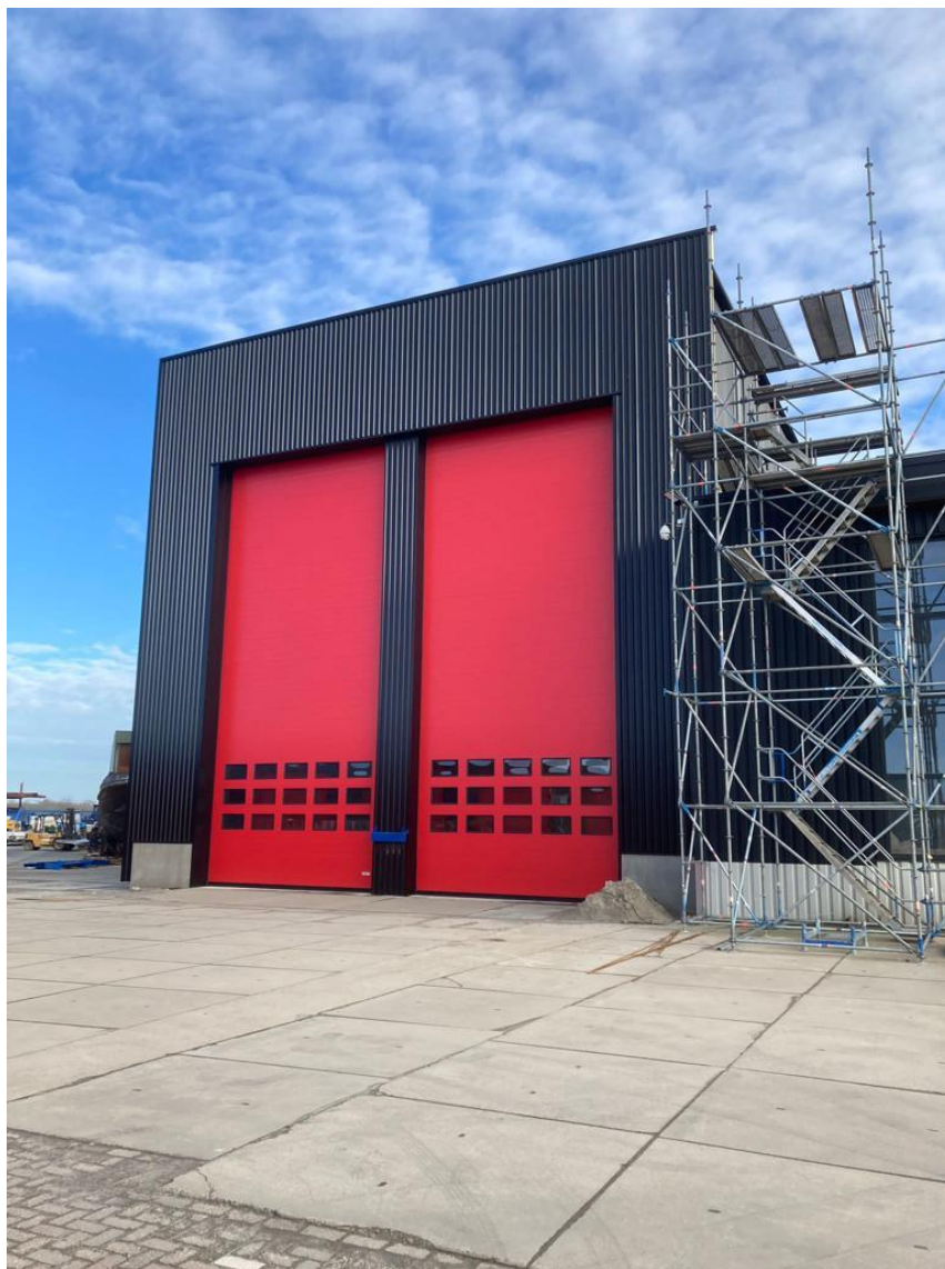
The new production facility at N. Dijkstra in Harlingen, where all of the RV Wim Wolff's hull sections will be joined together. ©FH
