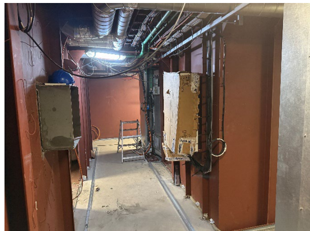
Cabin installation work
