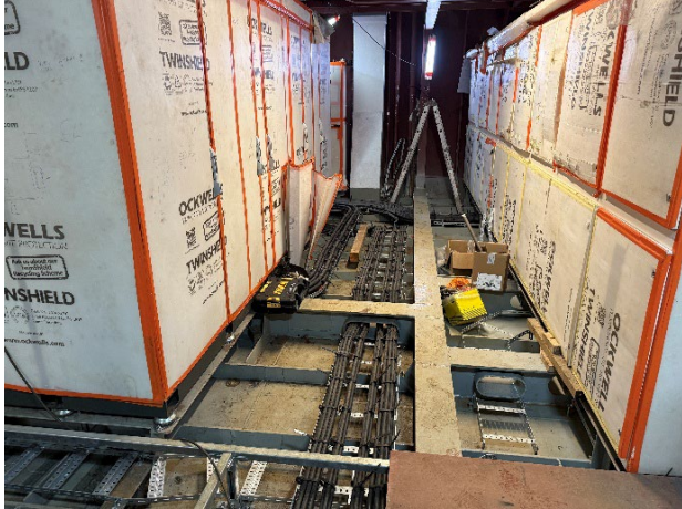
Installation work in the circuit box room.
