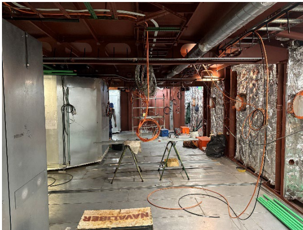
Work on the E-deck (crew).
