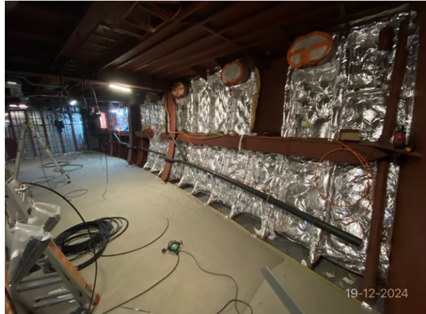
Concrete deck treatment on the F-deck and insulation against the outer hull.
