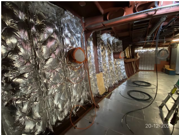
Insulating the cabins
