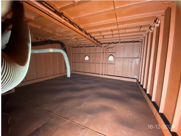
Sandblasting and painting the cabins
