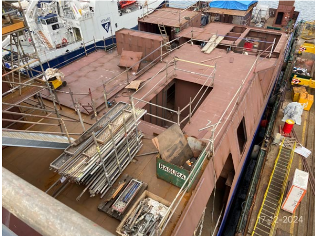
Sections AC 30 to AC41, seen from the wheelhouse
