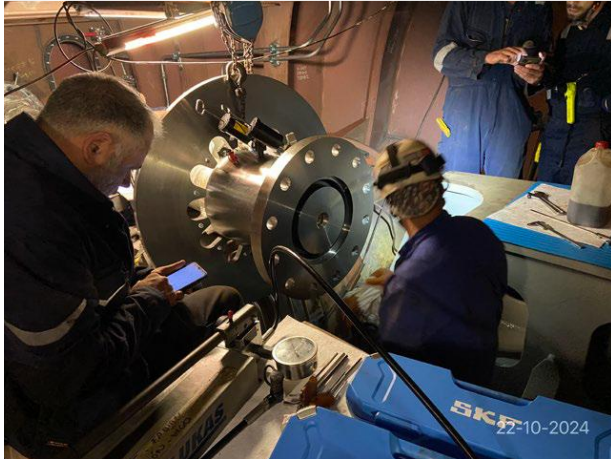
Pressurising the drive shaft coupling
