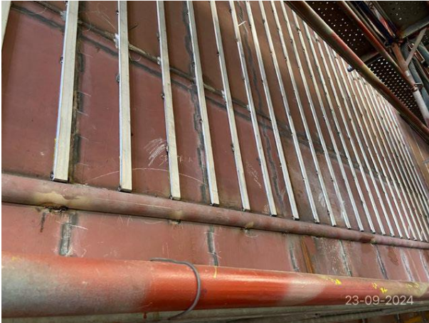
Preparations for fitting bolsters for the A-frame
