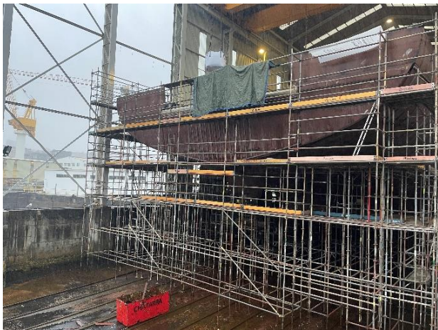
Front and rear views of the production facility.
