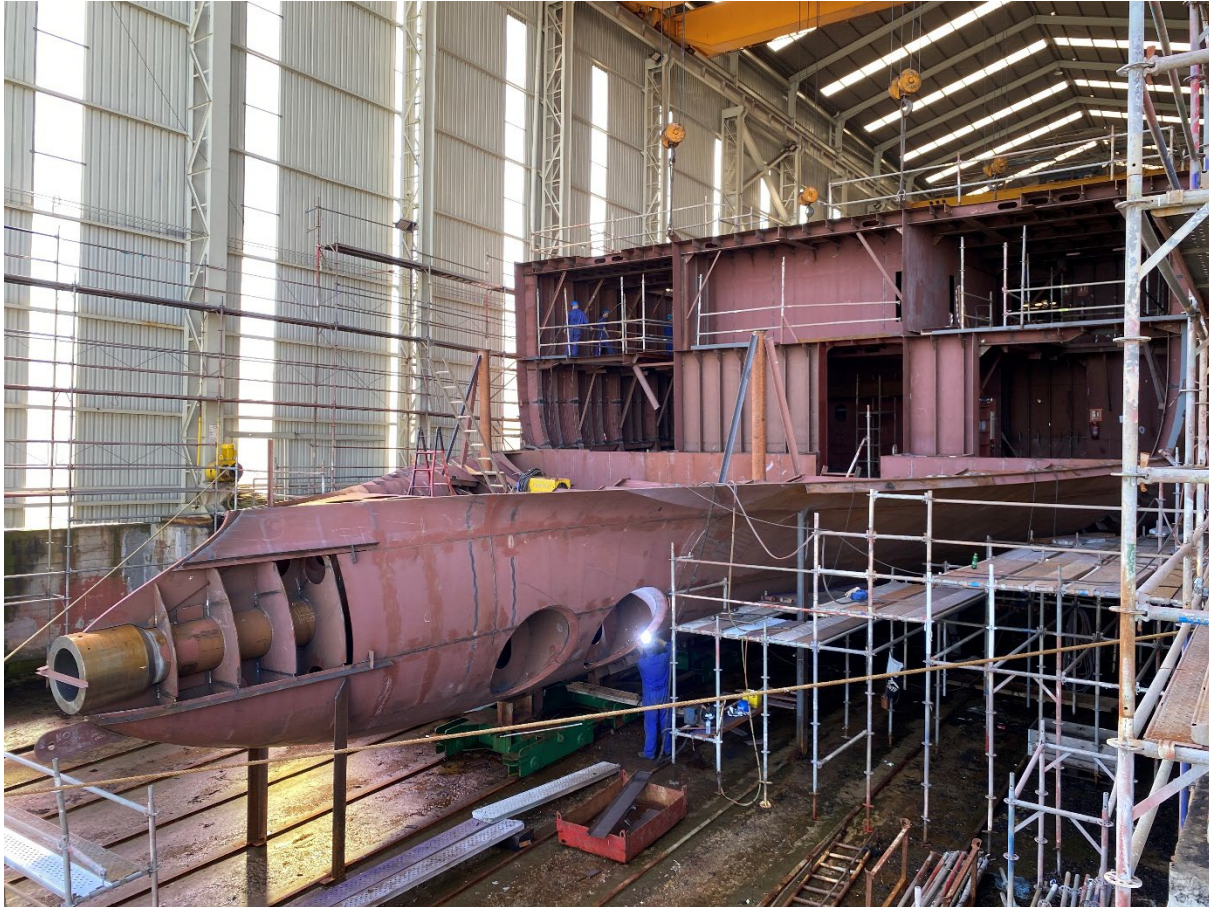
General overview of the production facility, with the drive shaft section.
