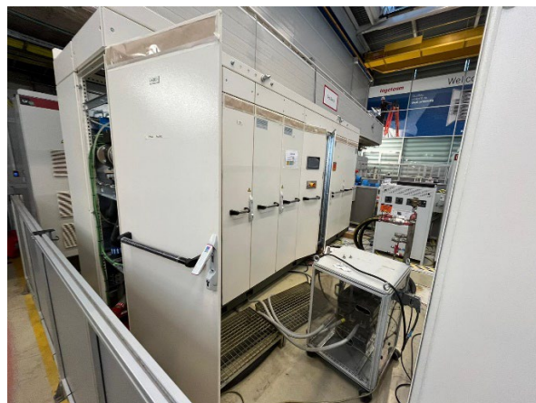
Delivery of the Multidrive in Bilbao
