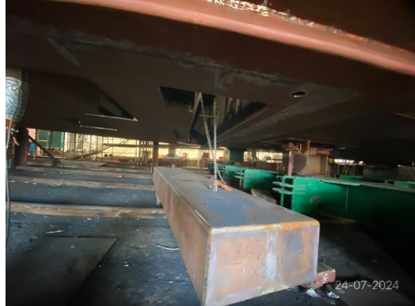
Multi-beam housing to be installed
