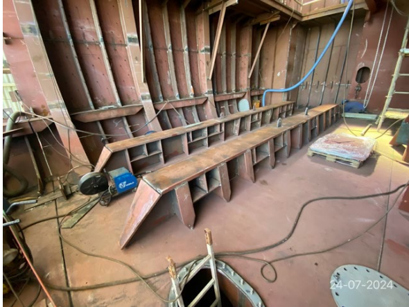
Engine mounts installed
