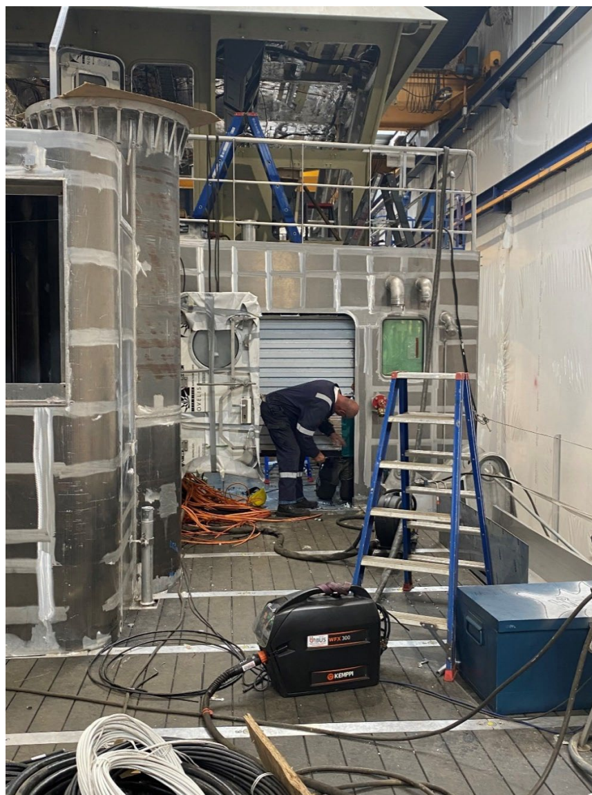
Assembly of the sliding between the wet lab and work deck
