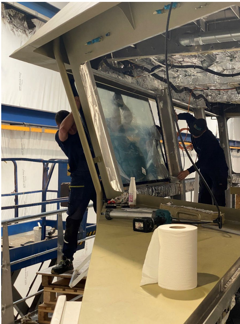
Mounting the portholes in the wheelhouse
