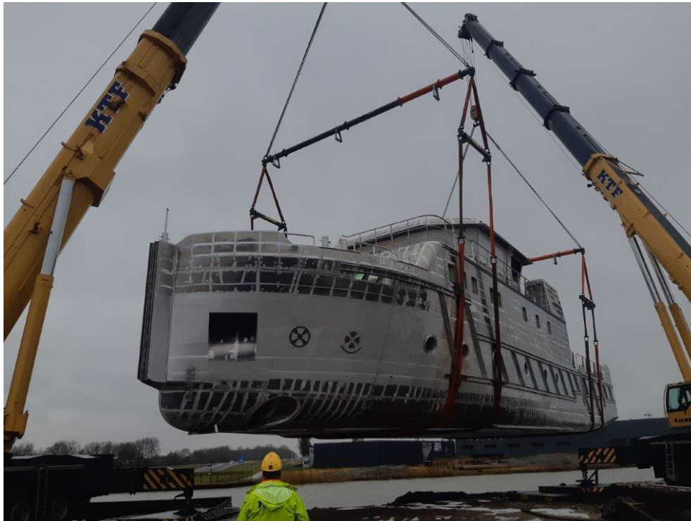
Crane lifting the hull. ©FH
