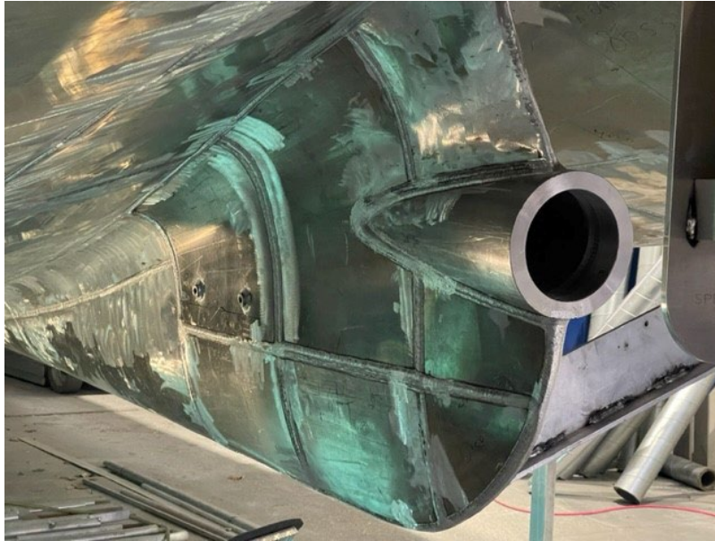
The stern tube for the drive shaft have been installed and aligned. The thickness of the stern tube is clearly visible in this photo. ©FH
