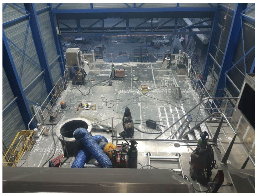
View of the work deck from the topside deck. ©PB
